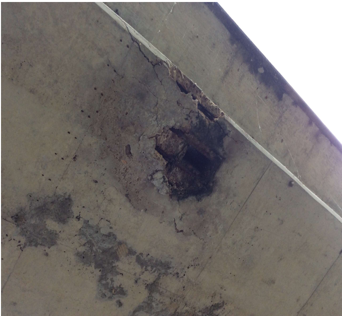
PHOTO 1 Description Typical spalled drain area.
